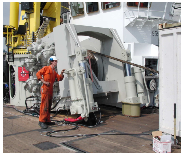
150t anchor handling winch being tested on-site.
