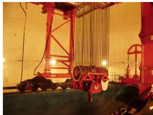
650 tons block and containerized gantry crane
