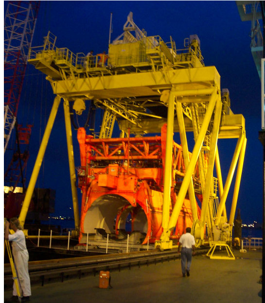
400Ts gantry crane with pipe handling frame
